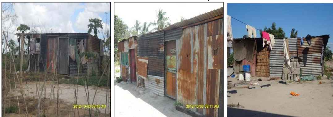
Plate 1: Some of the temporary huts used as shelter during the resettlement process, made of materials from demolished houses from previous settlements
