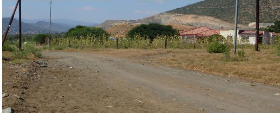
Above: The road in fair condition, with the Sefateng mine in the background
